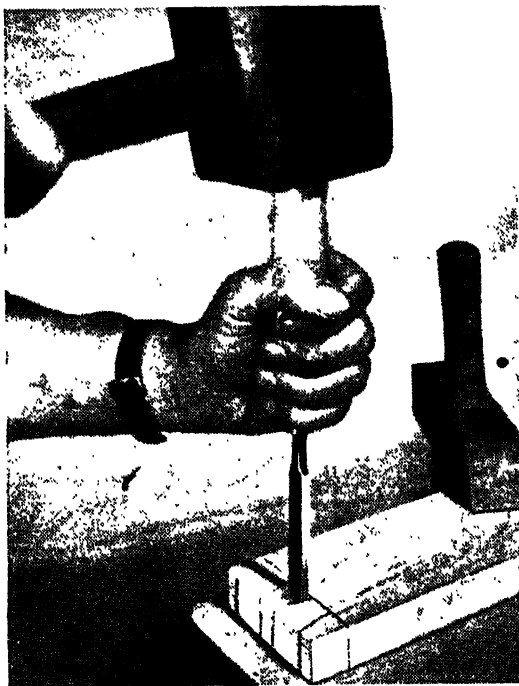
FIG. 22.—CHOPPING THE DOVETAILS. They are cut halfway through from each side.
